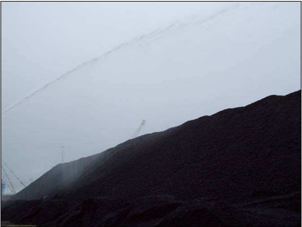
Fig 31. Polaris Rain Head operating in sequence at the Port of Blyth's 430m long Coal Compound. The system was designed and installed by HJ Banks Environmental Services in 2006.
