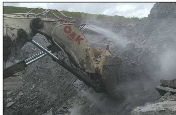
Fig 22. Spray Bars fitted to the excavator bars
