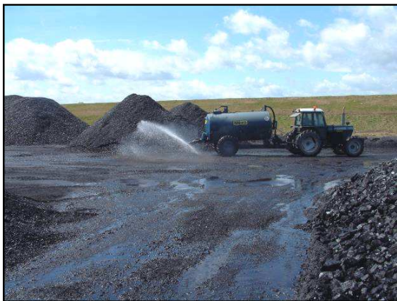
Fig 17. Using an agricultural tractor and bowser is effective on smaller sites
