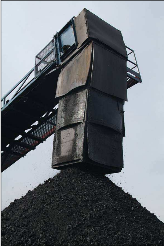
Fig 27. Dust Chute – fitted to the crushing plant at Delhi Surface Mine
